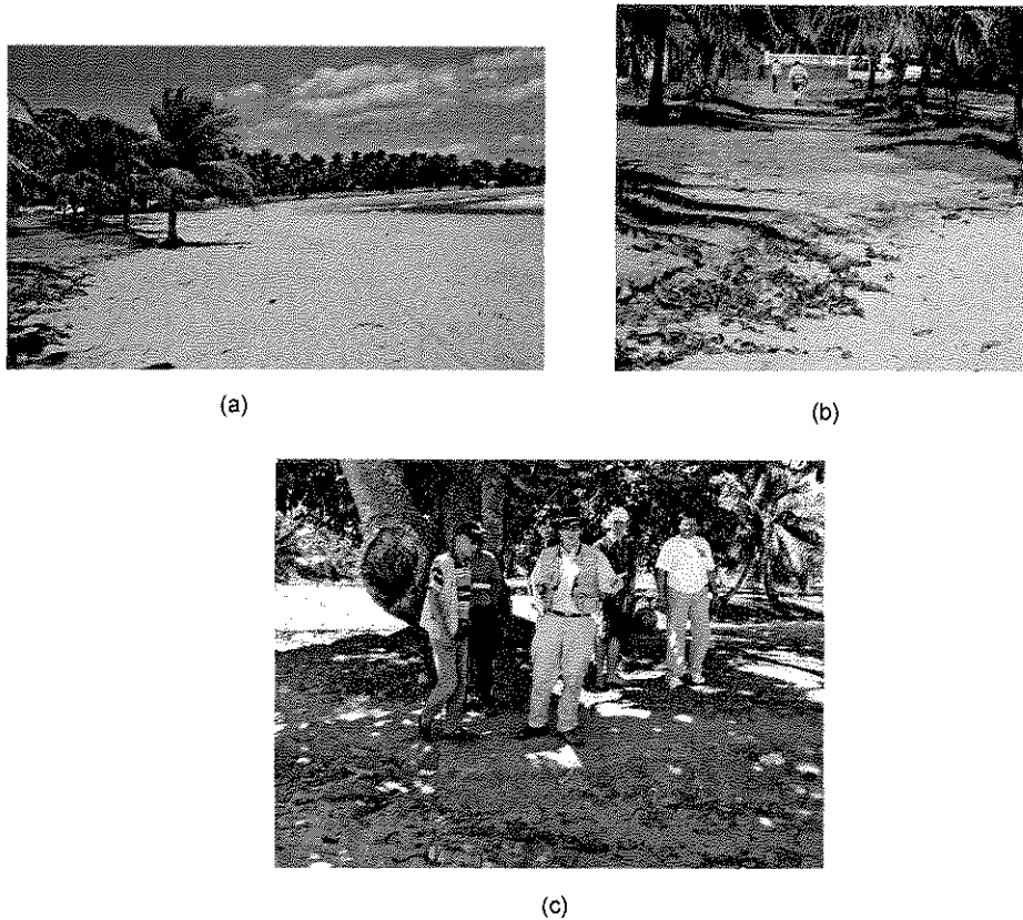
Figure 3. Scouring of a road along Ampandrozonana Beach in Sambava (Site 6). (a) General view of the beach, with the eroded road segment to the left, 71 m from the water line. (b) and (c) Close-up of the scouring. Note the advance of the beach, identified by sand deposits, over the previous location of the road.
