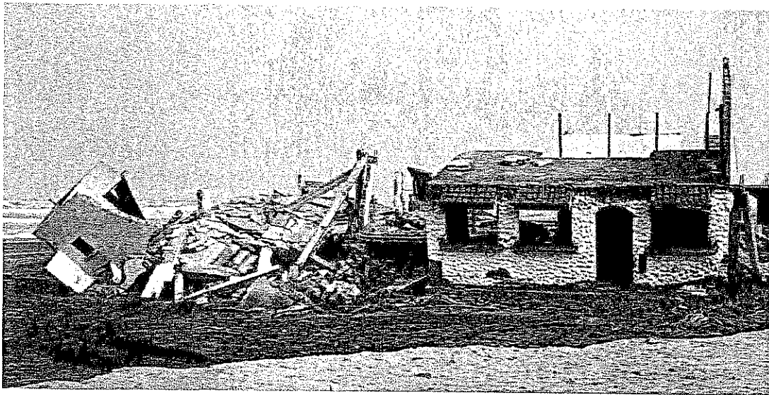
Figure 7-16. El Chorro discotheque built on filled river channel. Tsunami flow has undermined foundations of structure on the left.
