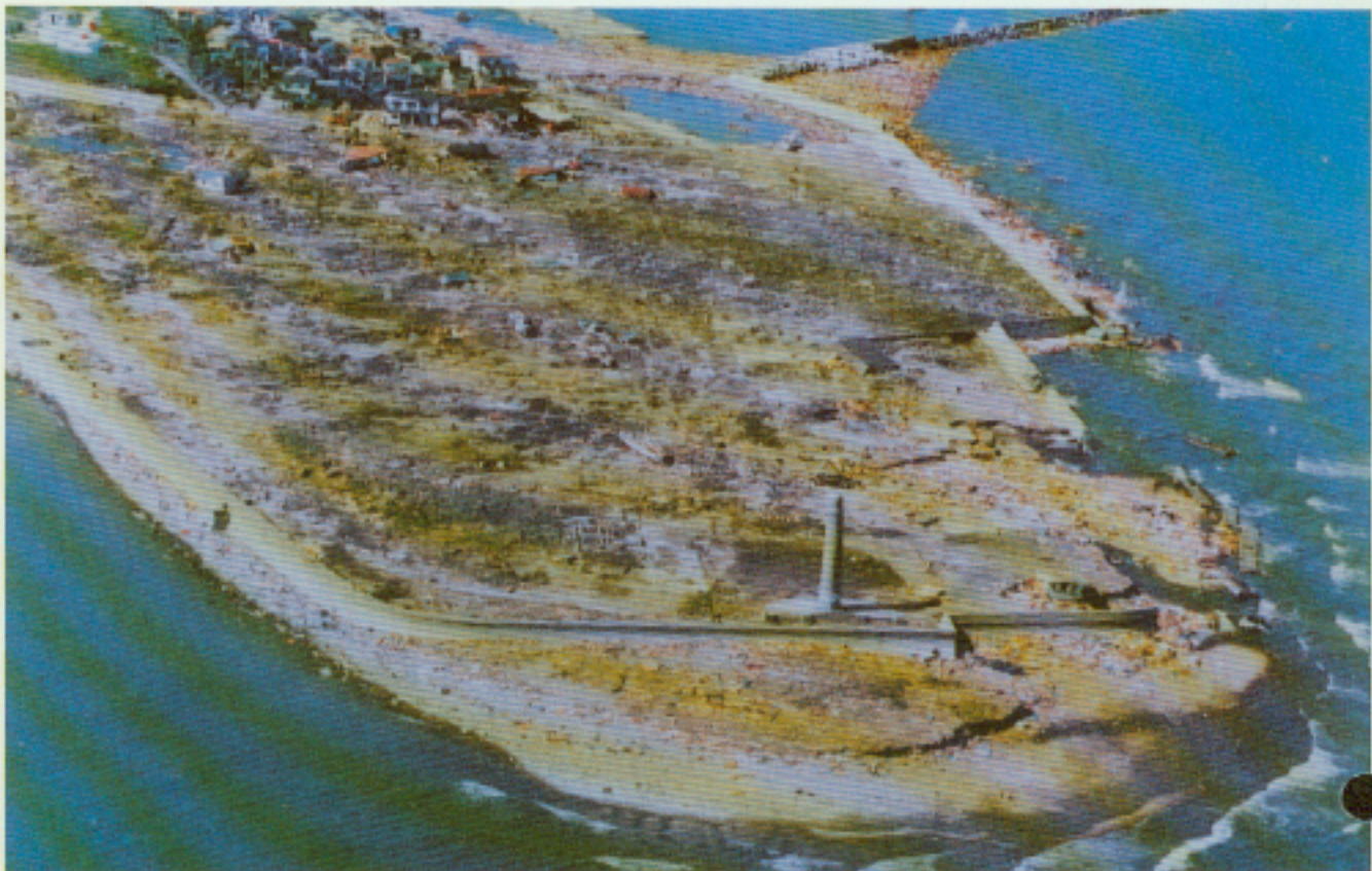
Figure 6 View of the southern tip of Okushiri island at Aonae, showing total destruction of the residential area to the South of figure 1. Note that the 4.5 m tall tsunami wall was overrun, and some of its sections even completely destroyed. (Courtesy of Y. Tsuji.)
