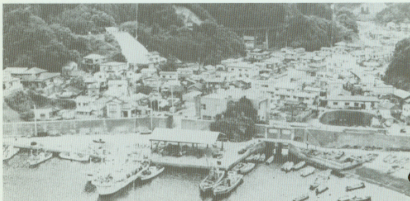
Figure 3 Example of tsunami wall in a typical fishing village (Ryoshi) along the Sanriku coast of Japan. Note the two groups of gates which allow traffic (vehicular — open at left; boat — closed at right), and which can be closed in case of a tsunami warning. The car near the left gate gives the scale: the wall is approximately 6 m tall.
