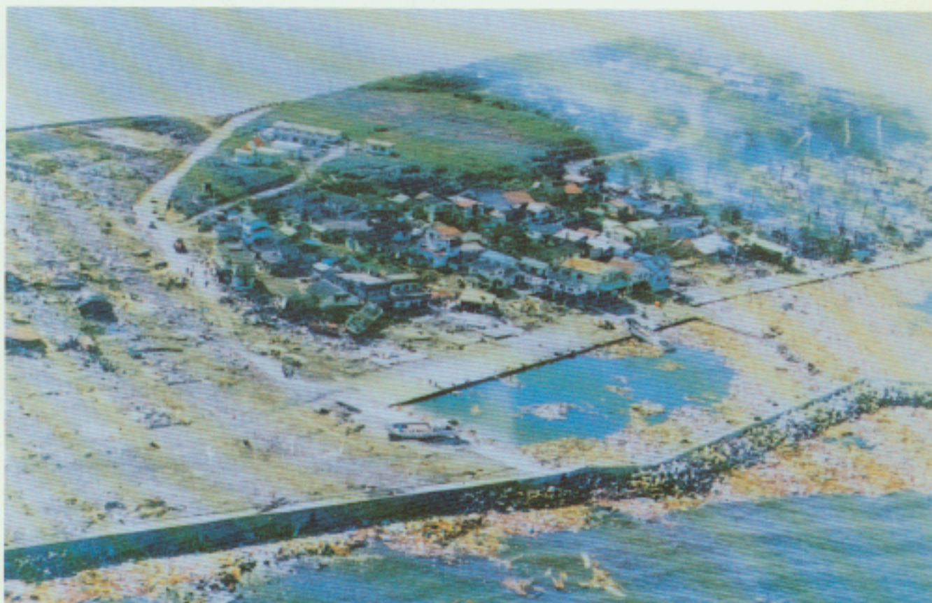
Figure 1 View of the small town of Aonae, on the island of Okushiri, Japan, in the aftermath of the Japan Sea tsunami of 12 July 1993. Note the devastation wrought on the island by the tsunami wave; all housing in the left part of the photograph has been destroyed and the rubble washed out in the harbour; note also the fishing boats carried inland and the fires, still burning in this next-day photograph. (Courtesy of Y. Tsuji.)
